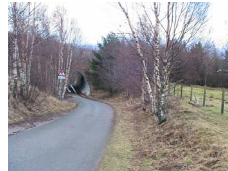
Fig. 11 : View east towards underpass
